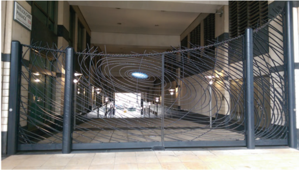
The works aren't always obvious. This gate designed by jeweller Katy Hackney has a celestial feel to it.
